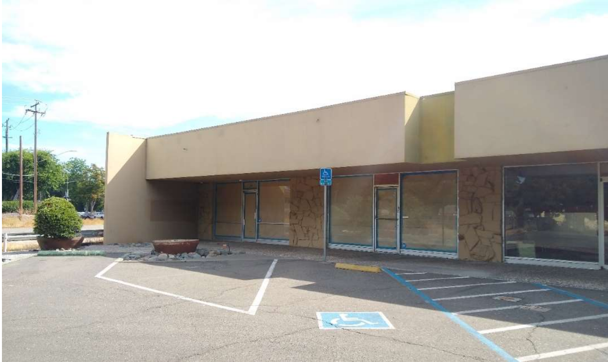
North end of west (primary) façade, ESA 2022.
